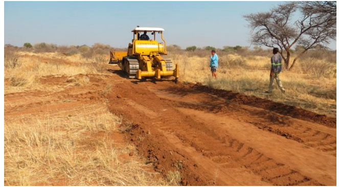
Figure 3: A line is ripped where soil dug from the ditch will be heaped to key in the bund to better secure it with the ground below.
