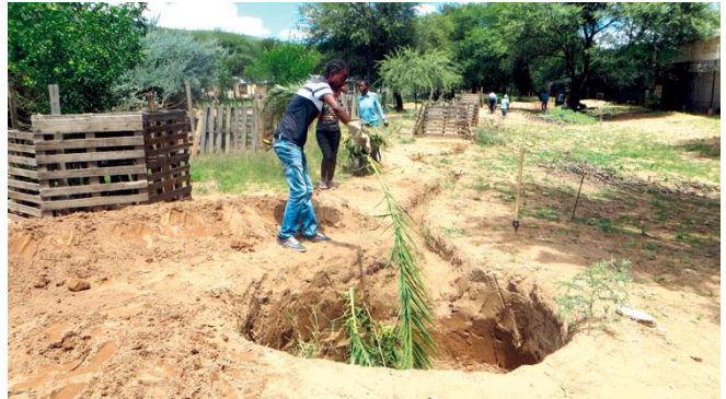
Figure 14: Organic material is thrown into a pit at the end of a contour ditch to improve fertility of infiltrating water.
