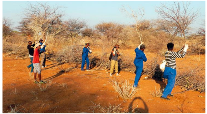
Figure 12: Branches are stacked to form a filter along the contour.
