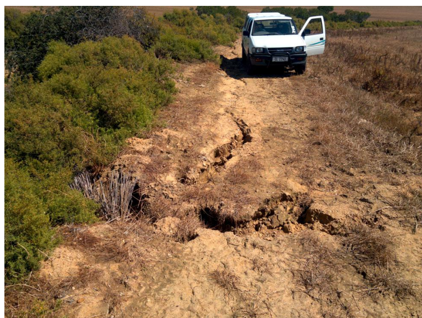
Figure 4: Bank gully expansion along farm dirt road
